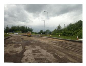
This week base course and binder has been laid between East Common Lane - the Wishing Well roundabout and between the swing bridge - northern layby averaging 1100 tonnes a day.
